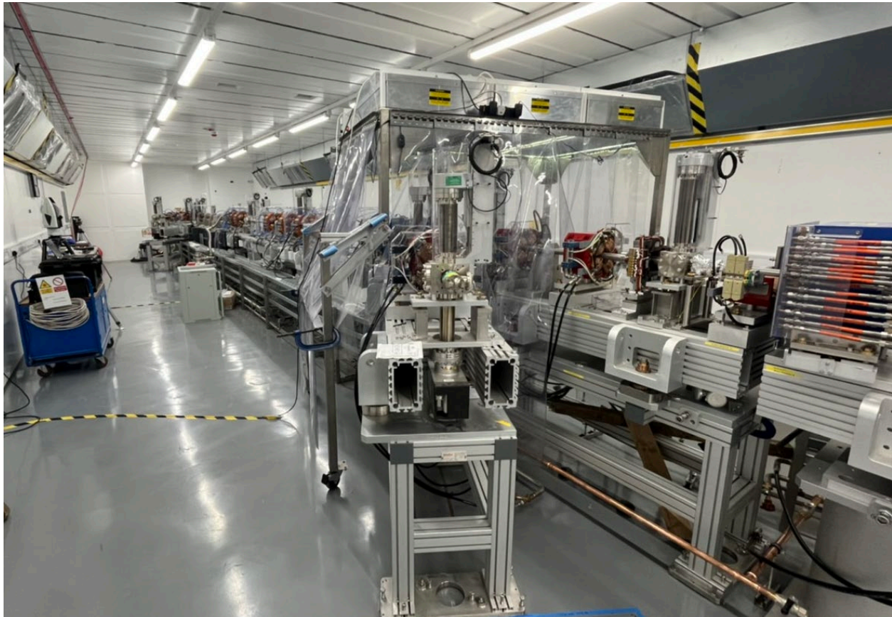
Figure 14- View of the CLARA facility (phase 2 construction).
