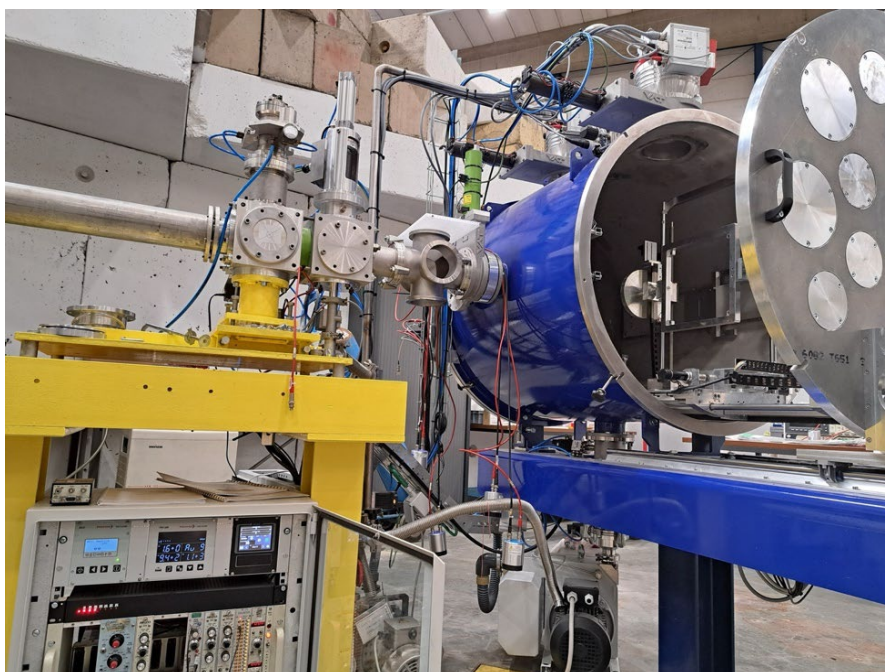
Figure 5: The end of the HIF beam line with the newly installed test chamber
